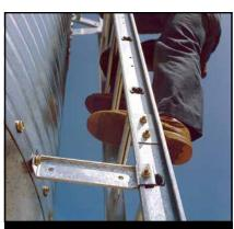
Sidewall Ladders have round rungs with a raised, non-skid surface and are permanently attached to the ladder rail for a hand-filling, secure grip.
